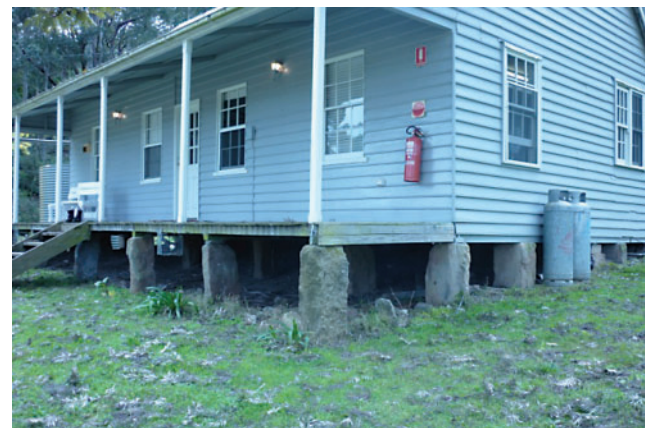
Fig. 1. The Musicians' Cottage, showing the sandstone piers and floodlight mounted underneath the veranda to the right of the stairs.
